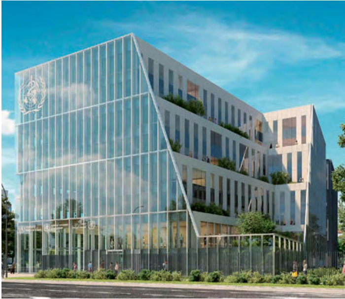
A digitally rendered mock-up of the WHO Academy's campus building, set for completion in 2024 in the heart of Lyon's bio-medical district.
