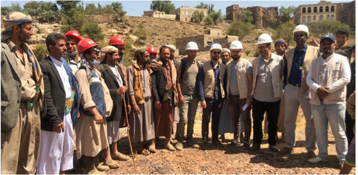
WFP and cooperating staff with the community committee overseeing the rehabilitation of a rural road in Sana'a Governorate.
